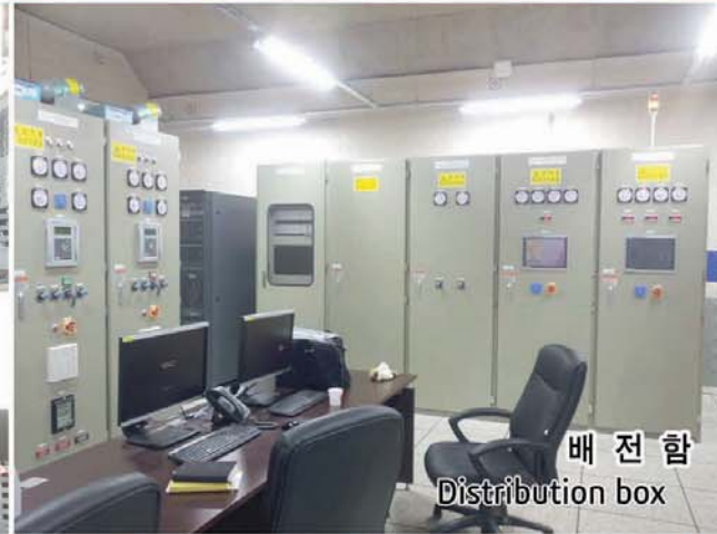
폐쇄형 배전반 Enclosed type distribution panel
