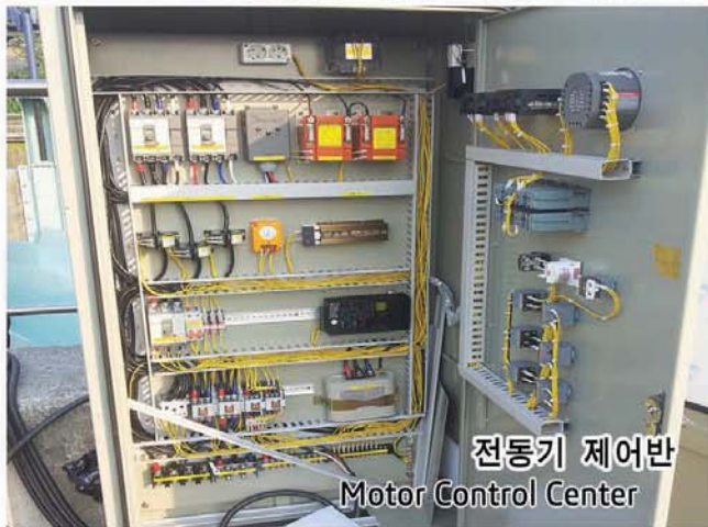
폐쇄형 배전반 Enclosed type distribution panel
