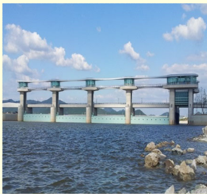
Shell Type Roller Gate
